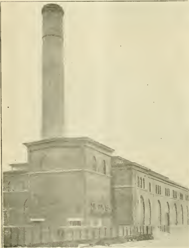
POWER-HOUSE FROM SOUTHEAST, SHOWING DUMPING CHUTES IN ASH TOWER, AND COALING TRACK.
